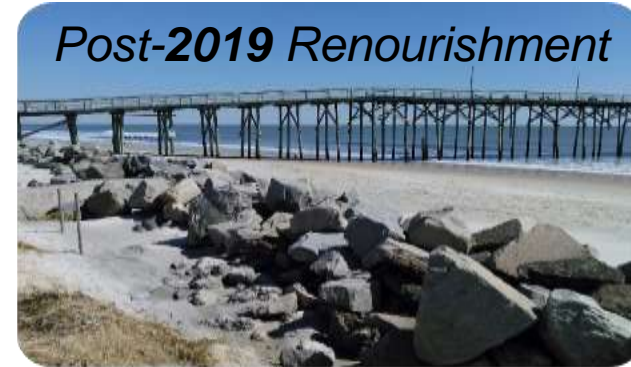
View Looking North
