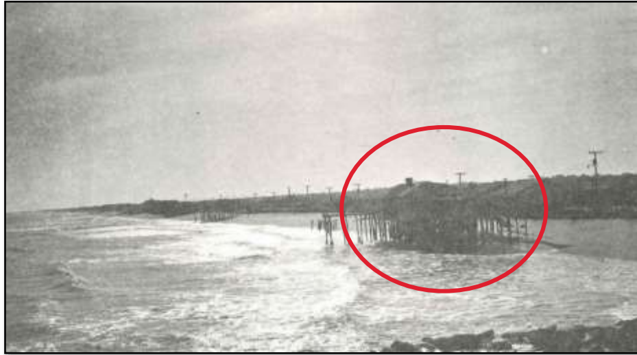
Carolina Beach Pre-Construction - 1964
