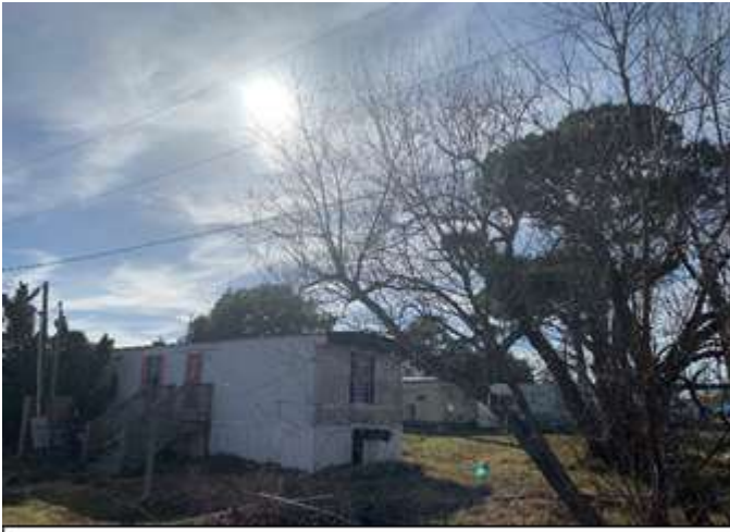
Demolition: 905 Basin Rd – 5 mobile homes
