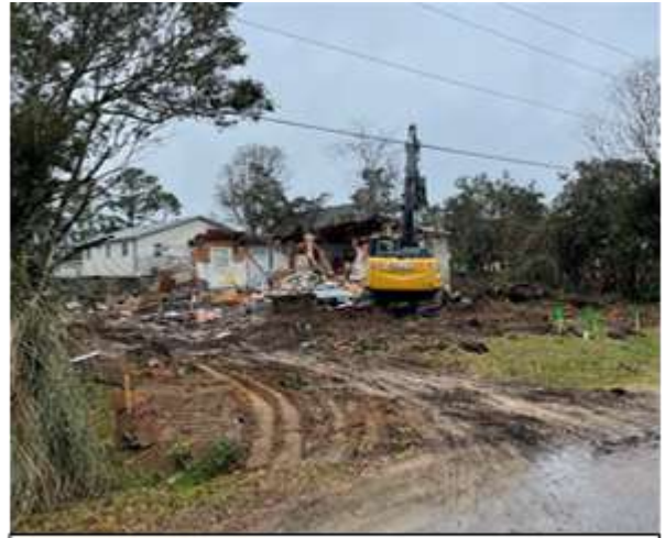
Demolition: 503 Greenville – single-family home
