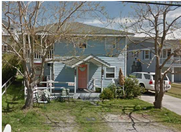
606 Canal Dr. – interior demo
