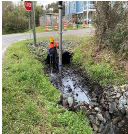
Cleaning check dams at 2 nd /Greenville Ave.
