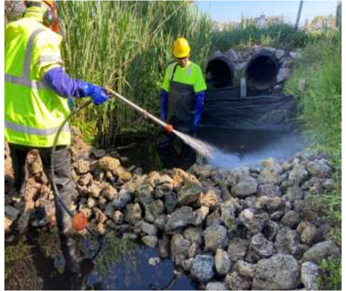
Crews cleaned check dams on Lake Drive
