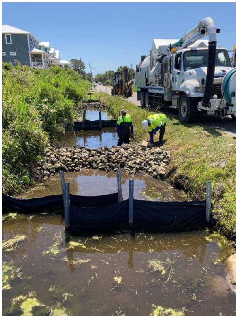
Crews cleaning filters on South Third St.
