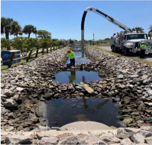
Crews cleaned check dams on Lake Drive
