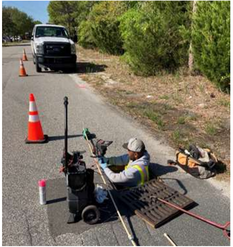
Crew inspecting stormwater pipes with camera at North 7 th St.
