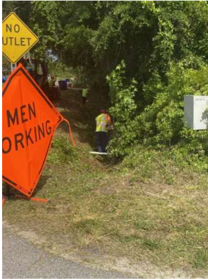
Crews perform stormwater drainage maintenance at Greenville Ave.
