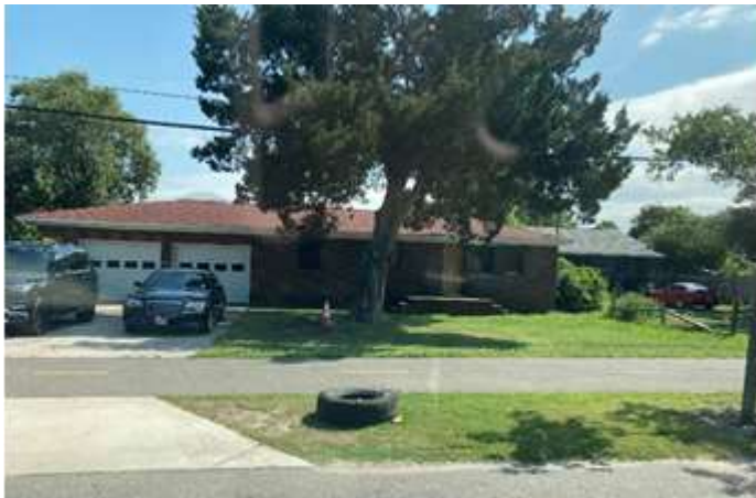
Demo: 413 Cape Fear Blvd. – House
