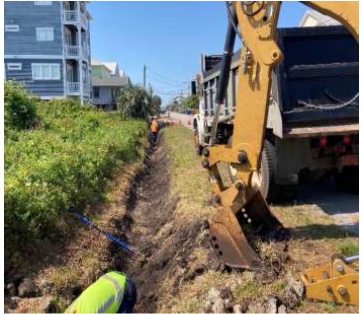
Crews reprofile ditches on Bowfin lane
