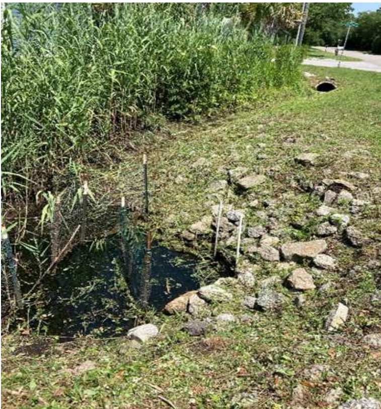
Crews clean out trash rack at St. Joseph St.
