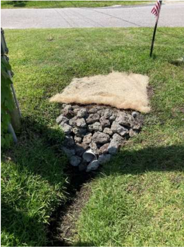
Crews upgraded stormwater pipe size on Atlanta Ave.
