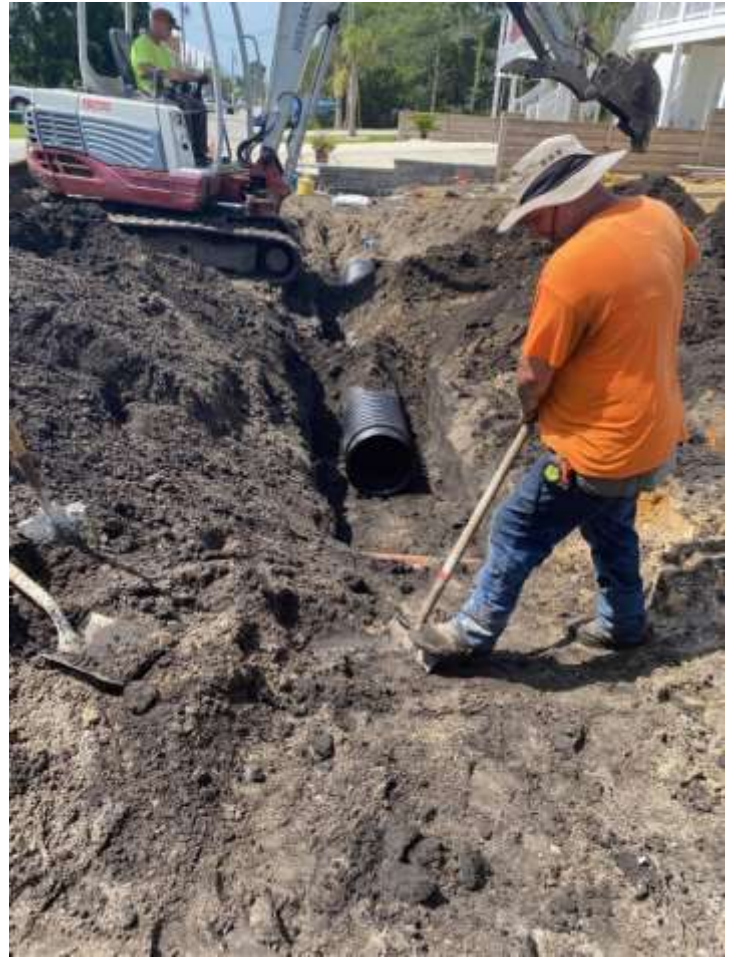
Contractors add stormwater system to 1400 block of Searay Lane
