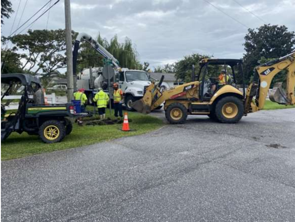
Crews repaired sinkholes on South Eighth St.
