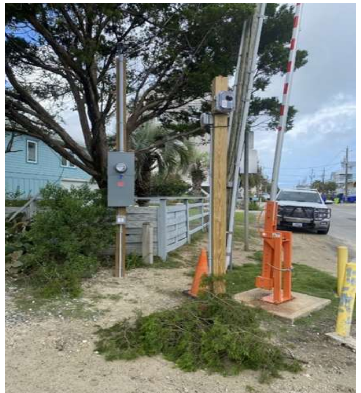
Power was connected at Starfish Ln. and Canal Dr. for flood monitoring sensors and camera. Users can scan the QR code and track flooding on their cell phones. Know when to avoid Canal Dr. and use CBA N as an alternate route to avoid driving in tidal water.
