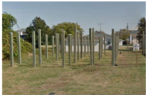
1211 Bonito/1507 Snapper – old pilings
