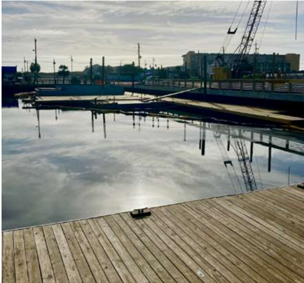
Marina Construction Progress
