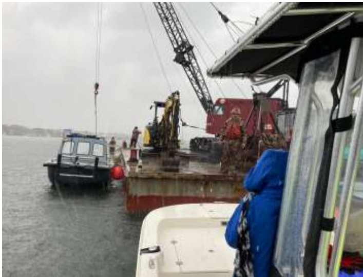
Mooring Field repairs
