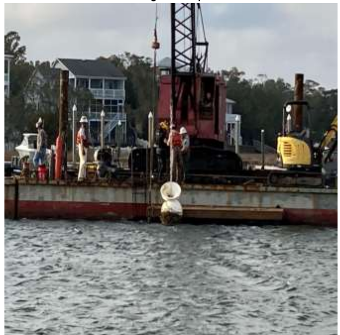
Mooring Field Repairs
