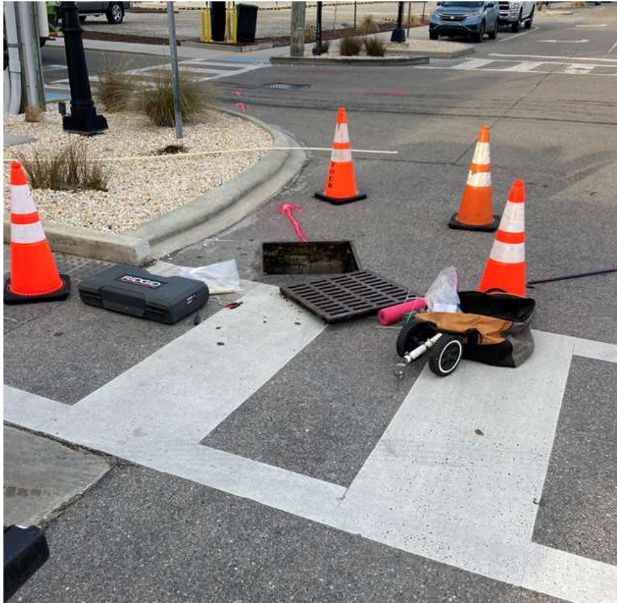
Crews map the stormwater system near Harper Ave.
