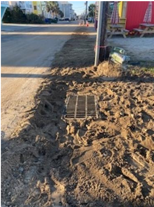
Contracted crews improve stormwater drainage on 900 block of CBA North.
