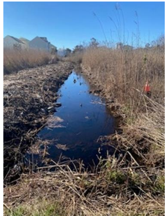
Contracted crews cleaned out South 2 nd St ditch.
