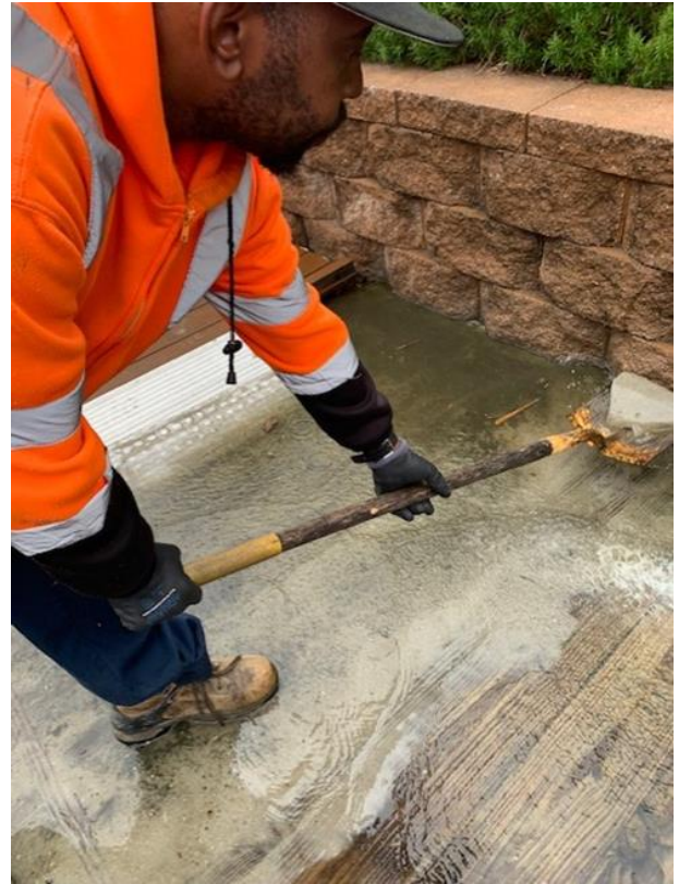
Town staff clean the boardwalk BMP
