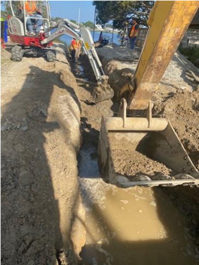
Contractor work started to upgrade the stormwater system at Starfish Lane.
