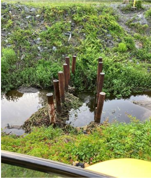
Town crews cleaned bollards at Henniker's ditch
