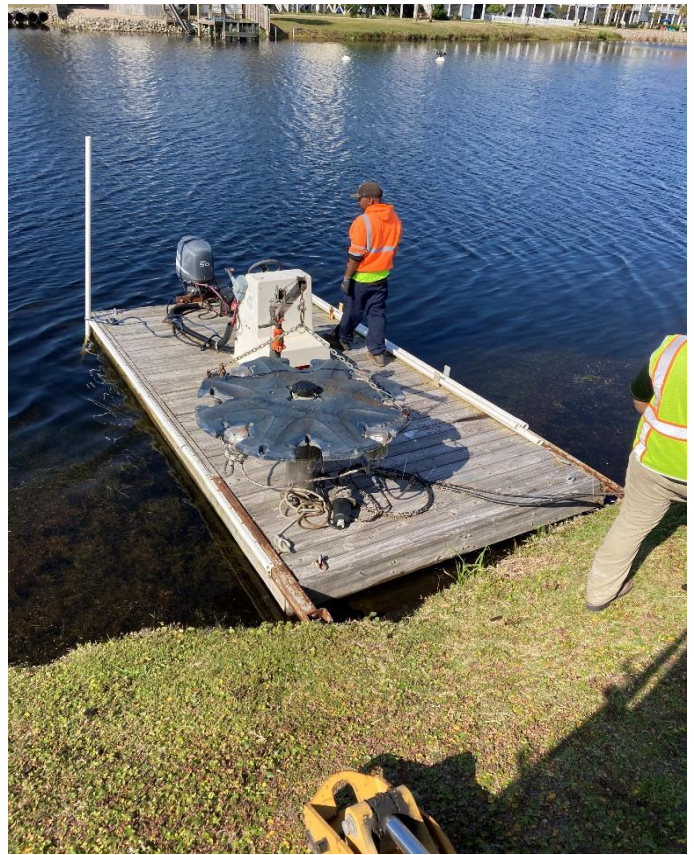
Town crews perform fountain maintenance at Lake Park.
