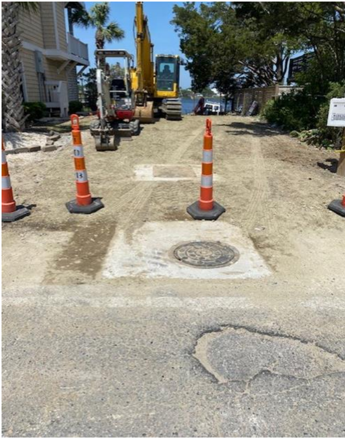
Stormwater upgrades completed at Start Fish Ln.
