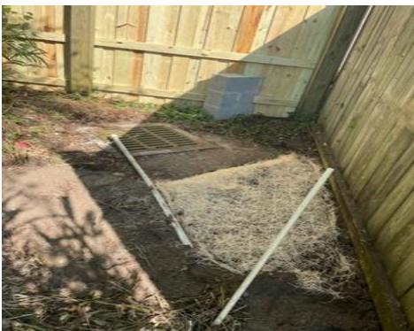
Crews completed stormwater repairs on Lewis/Teakwood Dr. easement.
