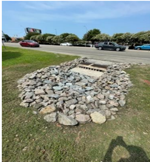
Town crews maintained the BMP on Access Rd.
