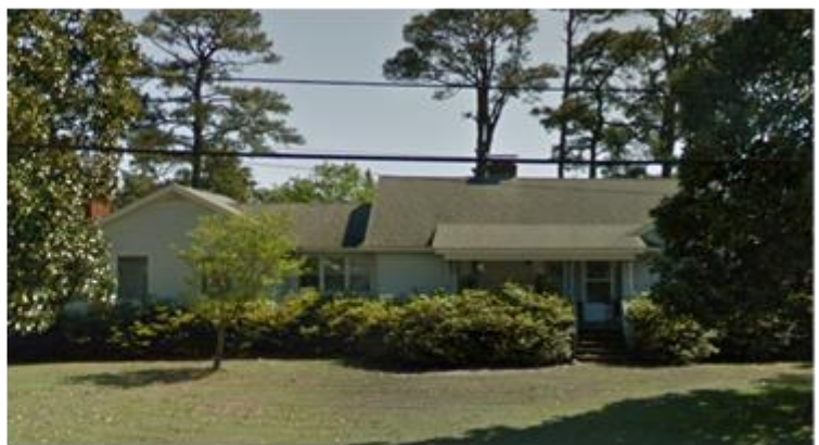
Demolition: 601 Cape Fear – single family home
