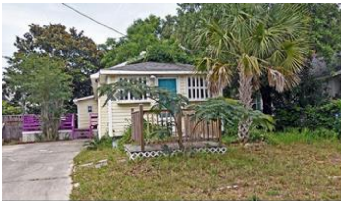
Demolition: 306 Wilson – single family home
