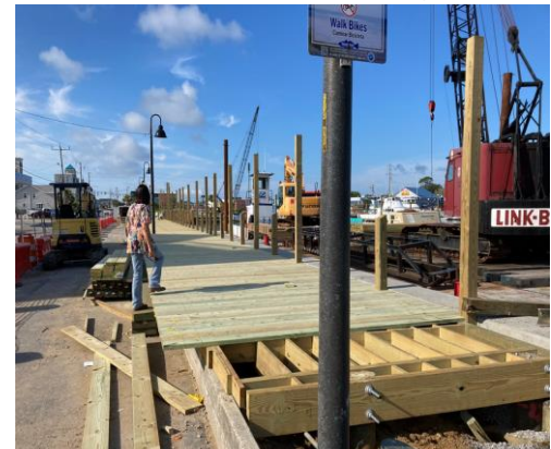
Marina construction progress
