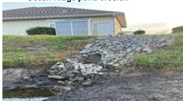
Crews repaired Ocean Ridge pond erosion
