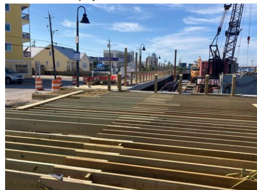
Marina project construction on east side
