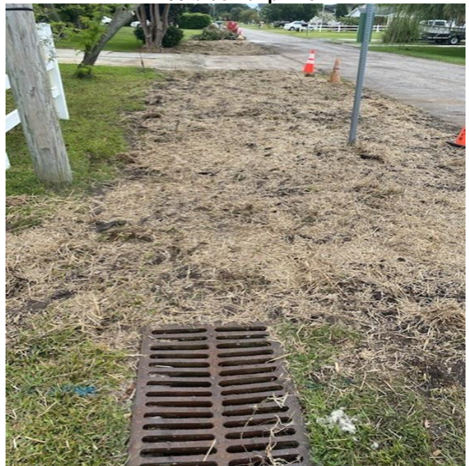
Contractor completed upgrade repairs on 1400 block of pinfish Ln.
