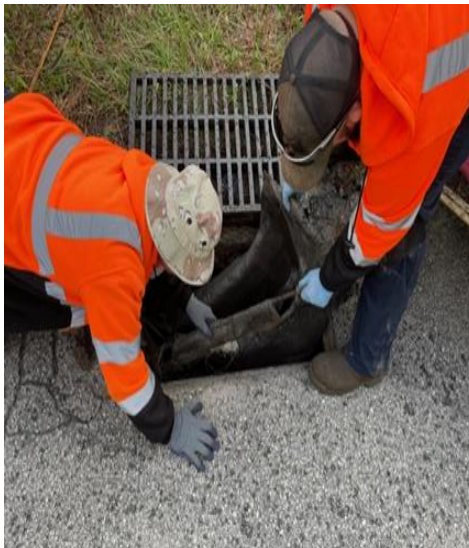
Crews Cleanout catch basin silt acks and camera stormwater pipes.
