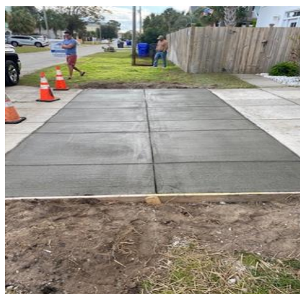
Crews finish sinkhole repair at 1404 Pinfish Ln.
