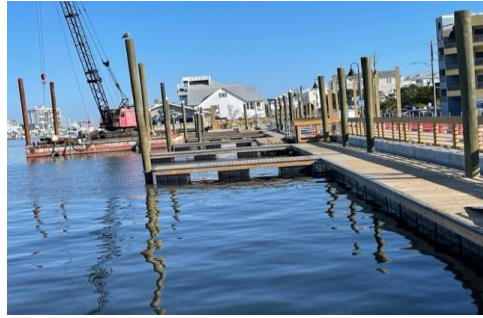
Marina Project: East side
