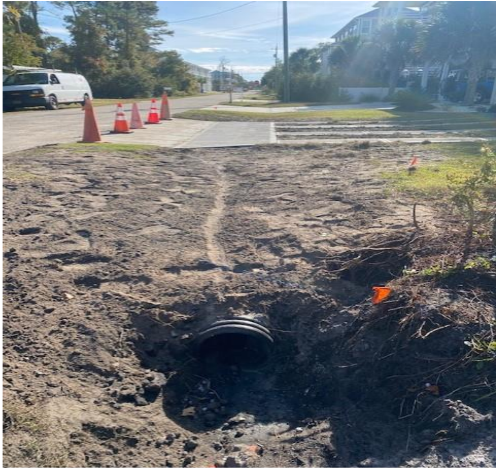
The contracted crew finished stormwater improvements at 1214 Mackerel Lane.
