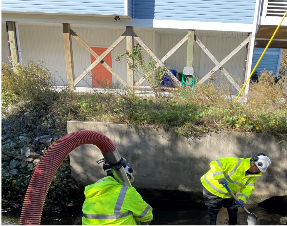
Crews cleaned out the inflow area at the Greenfield pump station.
