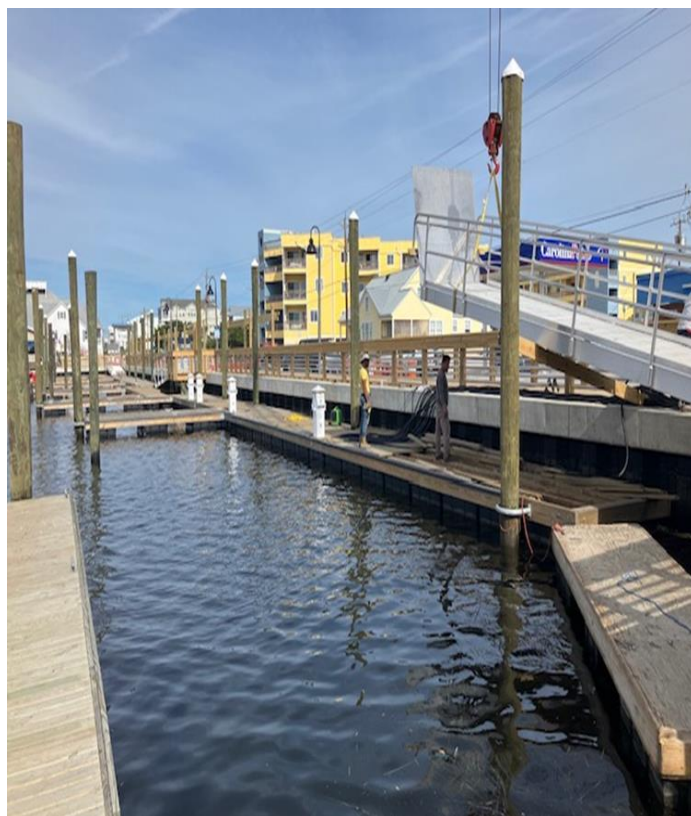
East side of Marina construction project
