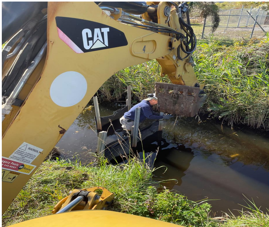
Crews remove turbidity curtains on Lake Drive.
