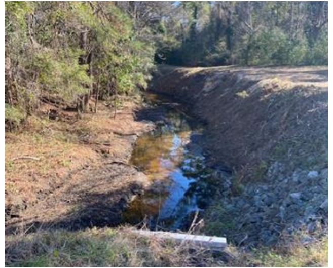
Contracted crews finished cutting Henniker's Ditch on the west side of Dow Rd.
