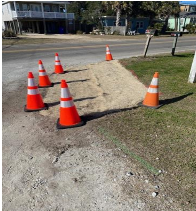
Town crews corrected drainage problem at 6 Tennessee Ave.
