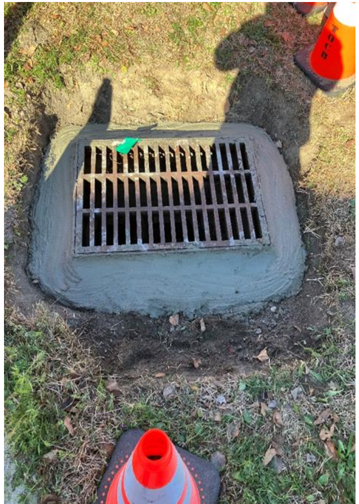
Crews repair frame and grate on Bonito Lane
