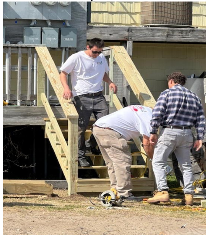
Contractor installing temporary stairs for electrical platform at Marina.
