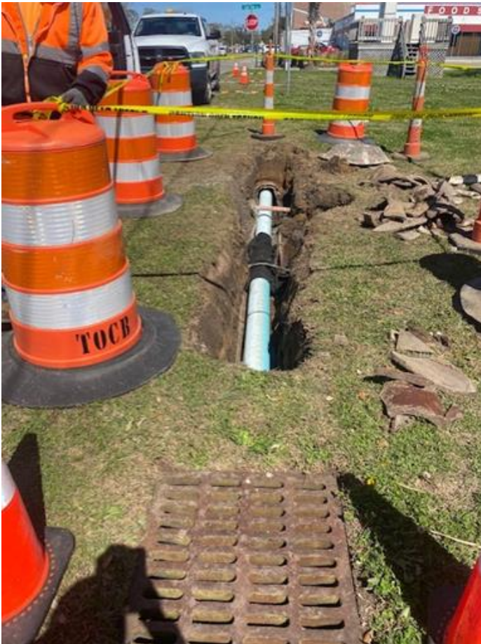
Stormwater crews repair sinkhole on south Third Street.
