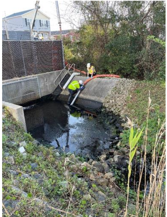
Crews clean out the Greenville Ave. pump station trash rack.
