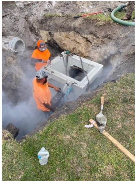
Stormwater addition to 700n block of Columbia Ave.
