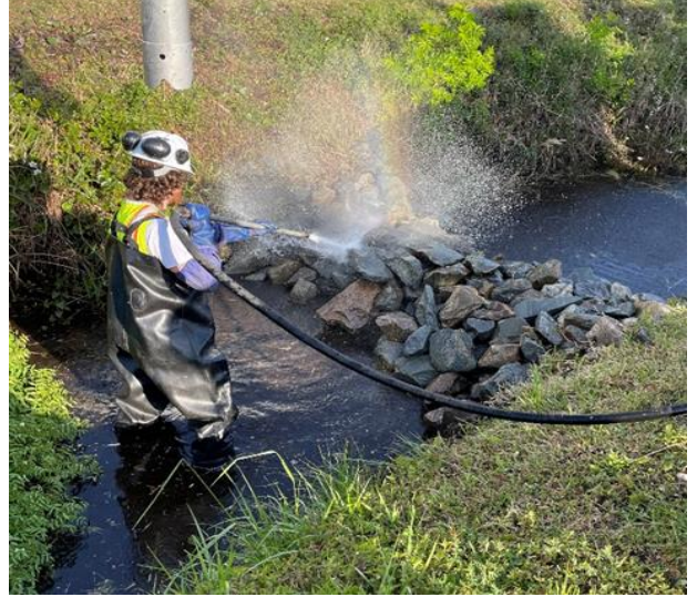
Crews clean check dams on South 2 nd Street.
