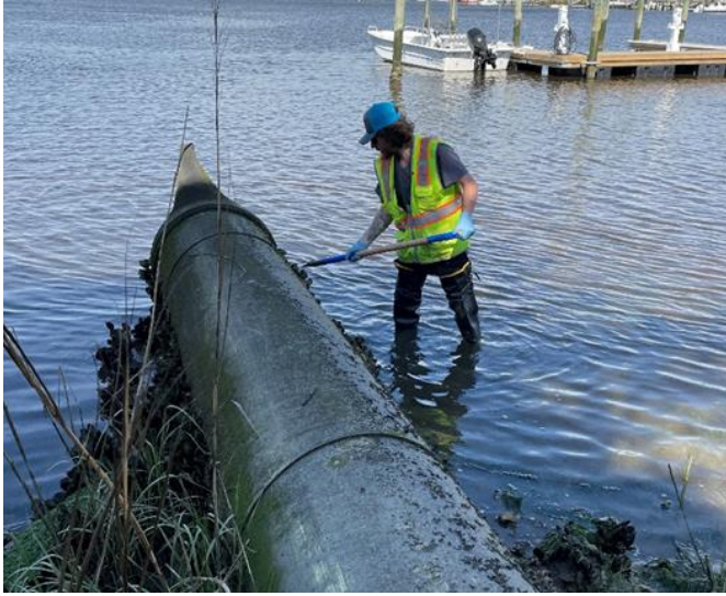
Crews clean and inspect outfall pipes.
