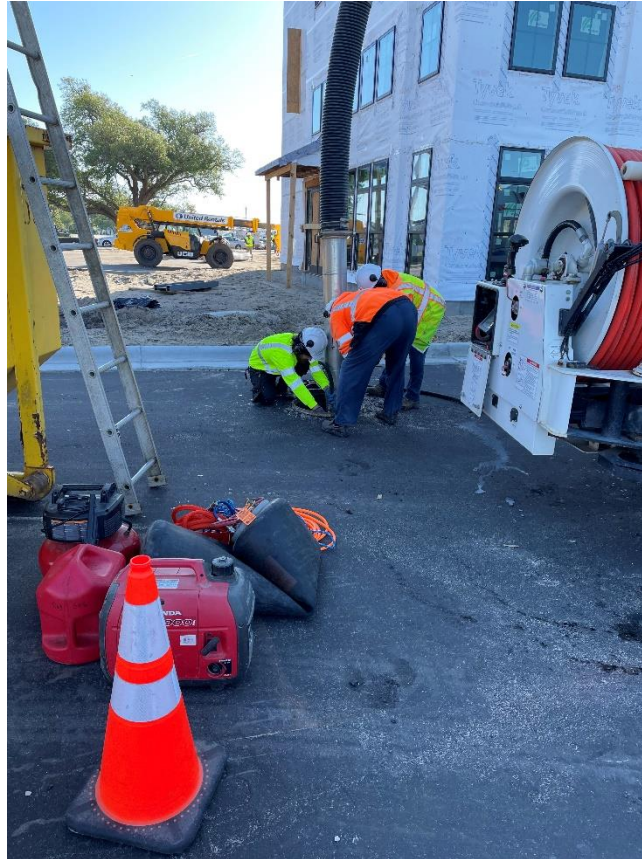
Crews clean out stormwater at Proximity.
