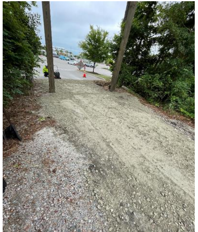
Crews repair driveway to Joseph Ryder Lewis Park.
