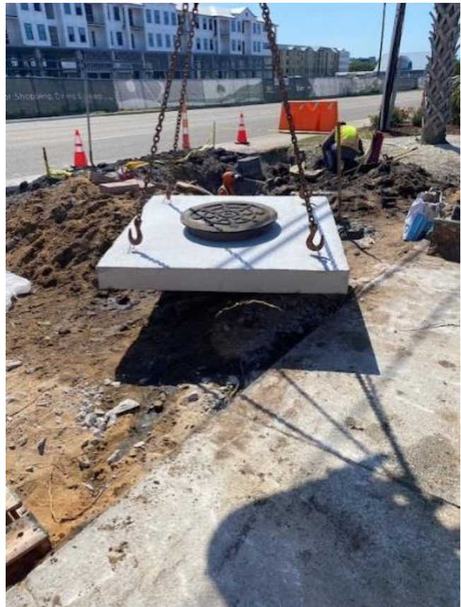
Contractors repair failed stormwater Pipes on North Lake Park Blvd.
