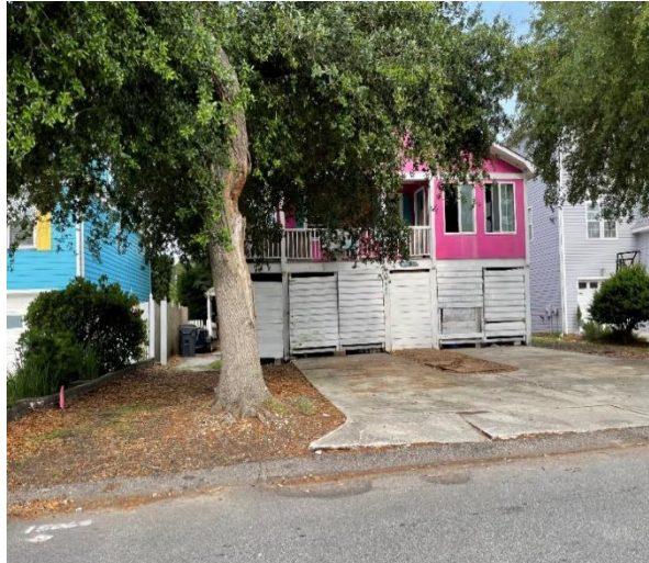
925 Carolina Sands Dr – Demo single-family House and rebuild through NC ReBUILD
