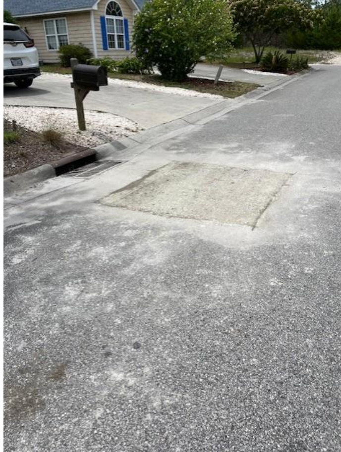
Stormwater crews repair sinkhole in Olde Mariners Way.
