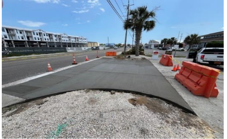
Contracted sinkhole repair on Lake Park Blvd completed.
