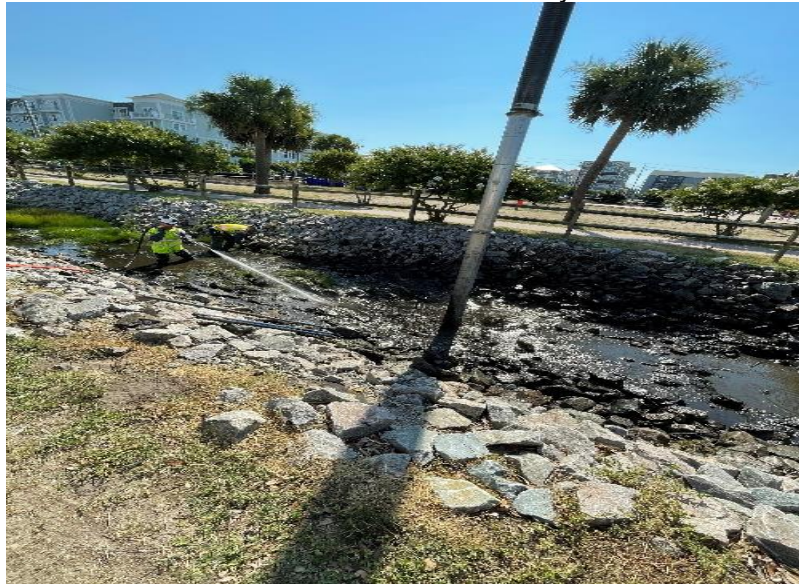
Stormwater crews clean the lake forebay at Atlanta Ave:
