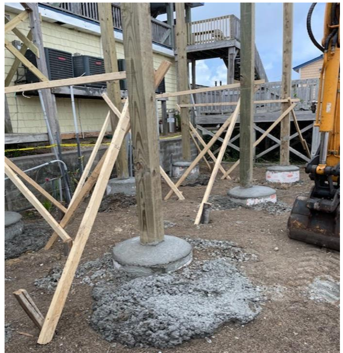
New pilings on electrical platform
