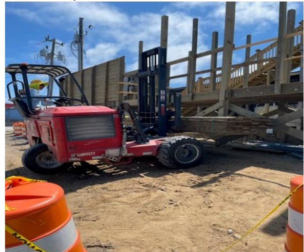
Electrical platform installation for west side.
