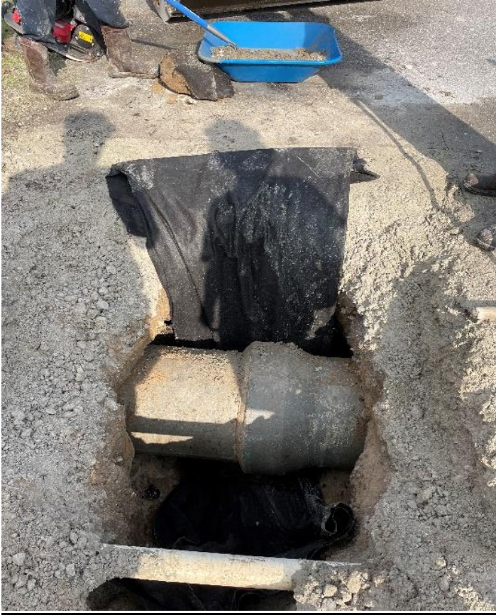
Stormwater crews repair sinkhole on Cape Fear Blvd.
