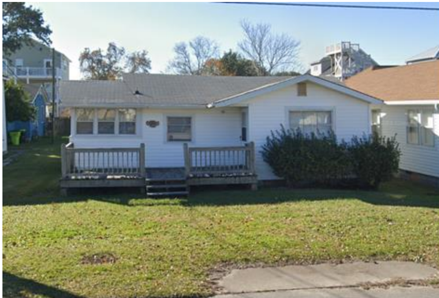
Demo: 309 Cape Fear Blvd. – House and Shed
