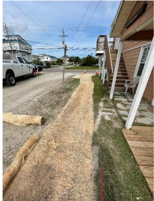
Crews work to improve drainage at Tennessee Avenue parking lot.
