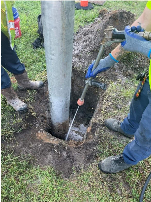
Crews repair sinkholes on the 1500 block of Mackerel Lane.
