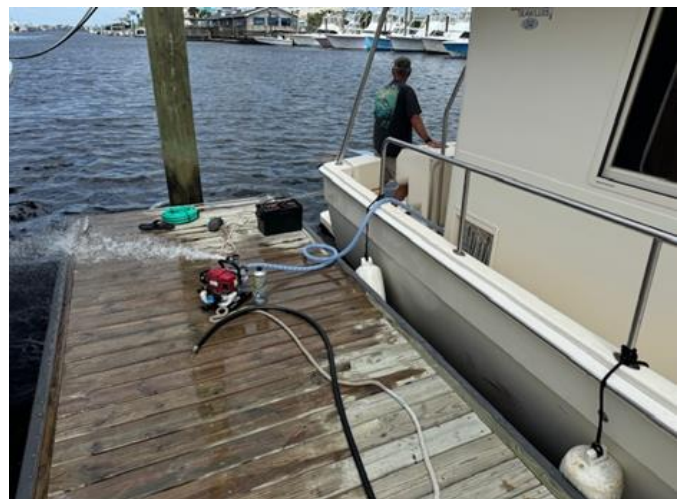
Harbor Master's gas powered pump in action
