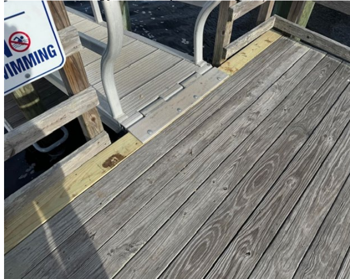
Dingy Dock repairs being made
