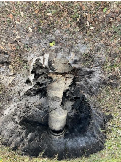
Stormwater crews repaired a sinkhole on Bonito Lane.
