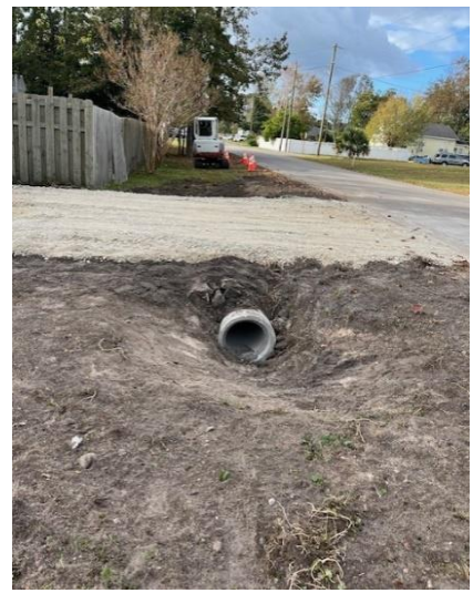
Contracted crews replace broken pipe and restore ditch at 6 th /Birmingham
