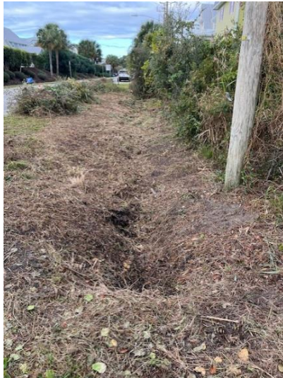
Stormwater crews clear ditch on Spencer Farlow Dr.
