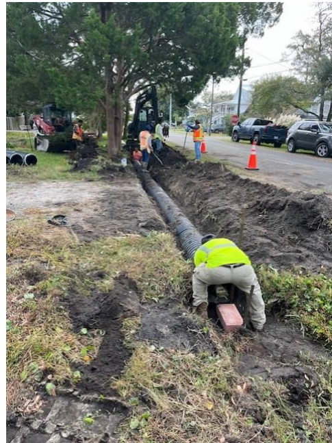
Contracted crews replace old stormwater pipes at South 5 th street and Birmingham Ave.
