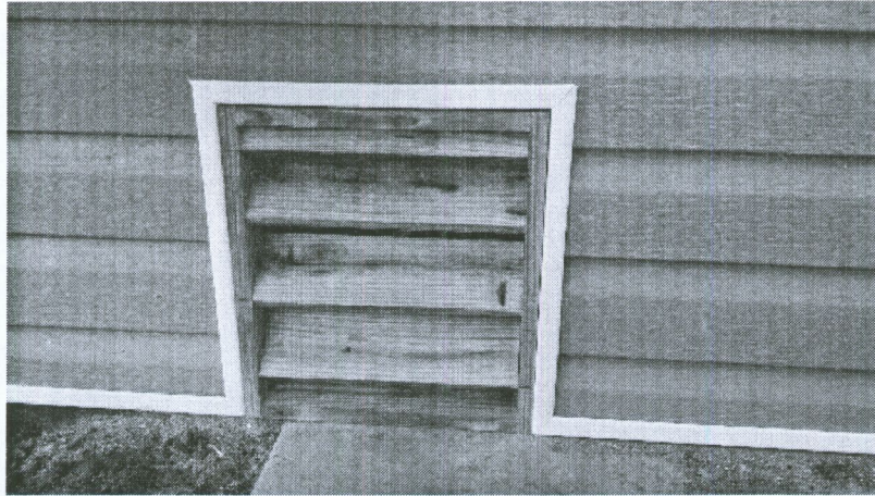
PHOTOS TAKEN SEPTEMBER 11, 2014 (VENTS INSTALLED AFTER INITIAL PHOTOS TAKEN)
