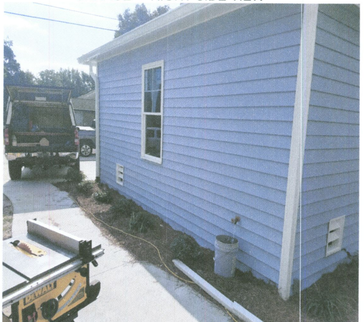
GARAGE - RIGHT SIDE VIEW
